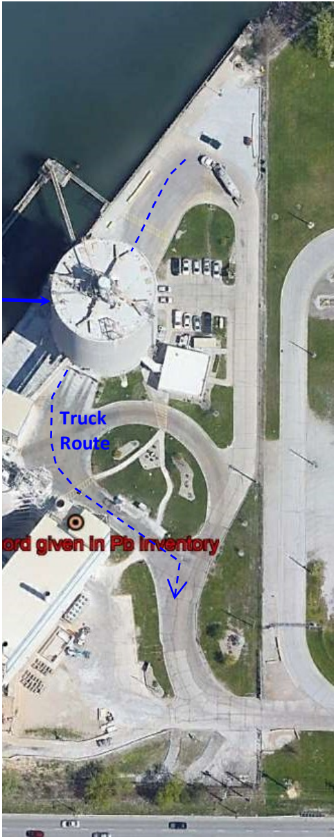
of Holcim US : - Chicago, Illinois
